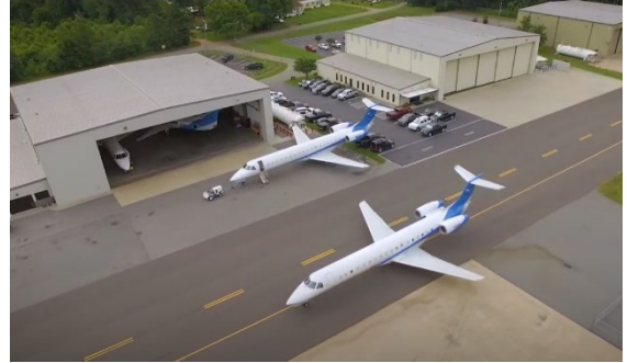
Figure 4: The Statesville Airport is an additional pathway into the region alongside Interstates 40 and 77
